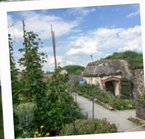
Up on the roof
